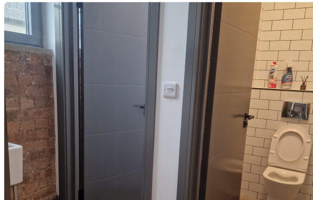
WC facilities Modern fit-out
