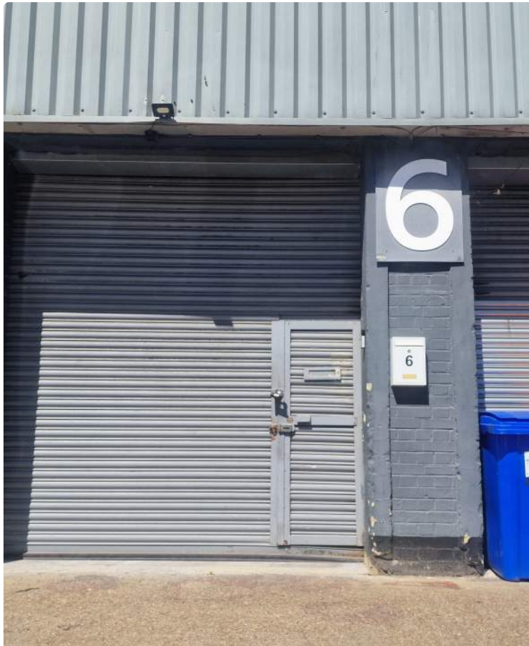
Unit 6 frontage Electric shutter access
